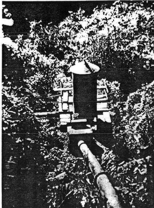
FIG. 1.2 Micro hydro plant installed in 1959 in Unduavi, Bolivia, with a capacity of 15 kW.
